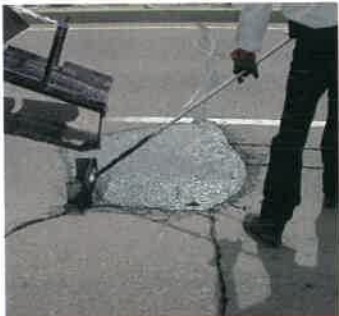
Pothole Repair
